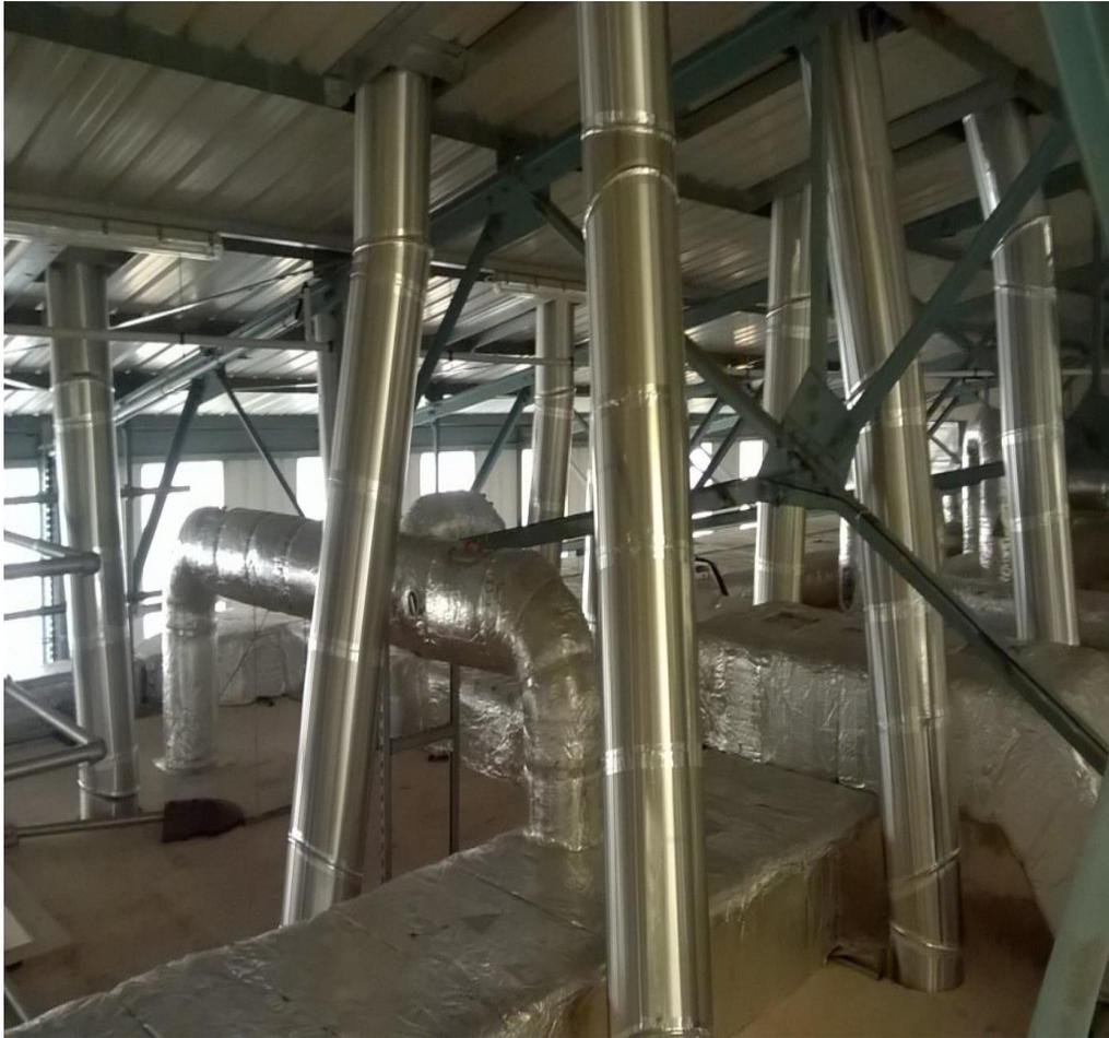
The Sun Pipes leading from Roof Domes to office ceiling Diffuser's
