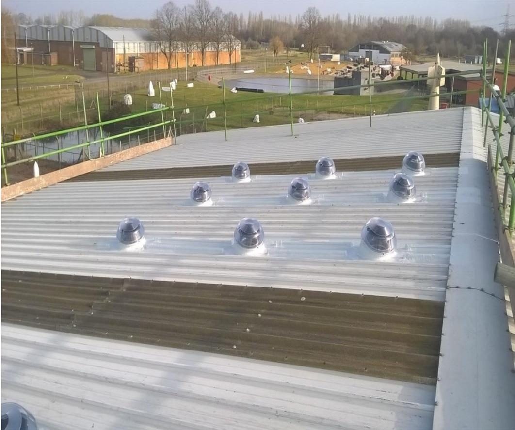
The Roof Domes of the Sun Pipes installed at building BCB001
